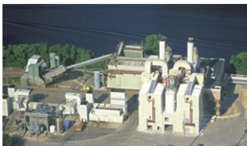
Xcel's WTE facility - French Island
