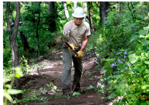
Trail Building at Landfill by Wiscorp
