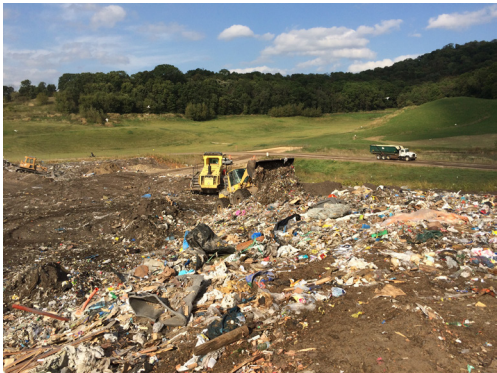
Phase VIII waste placement and compaction
